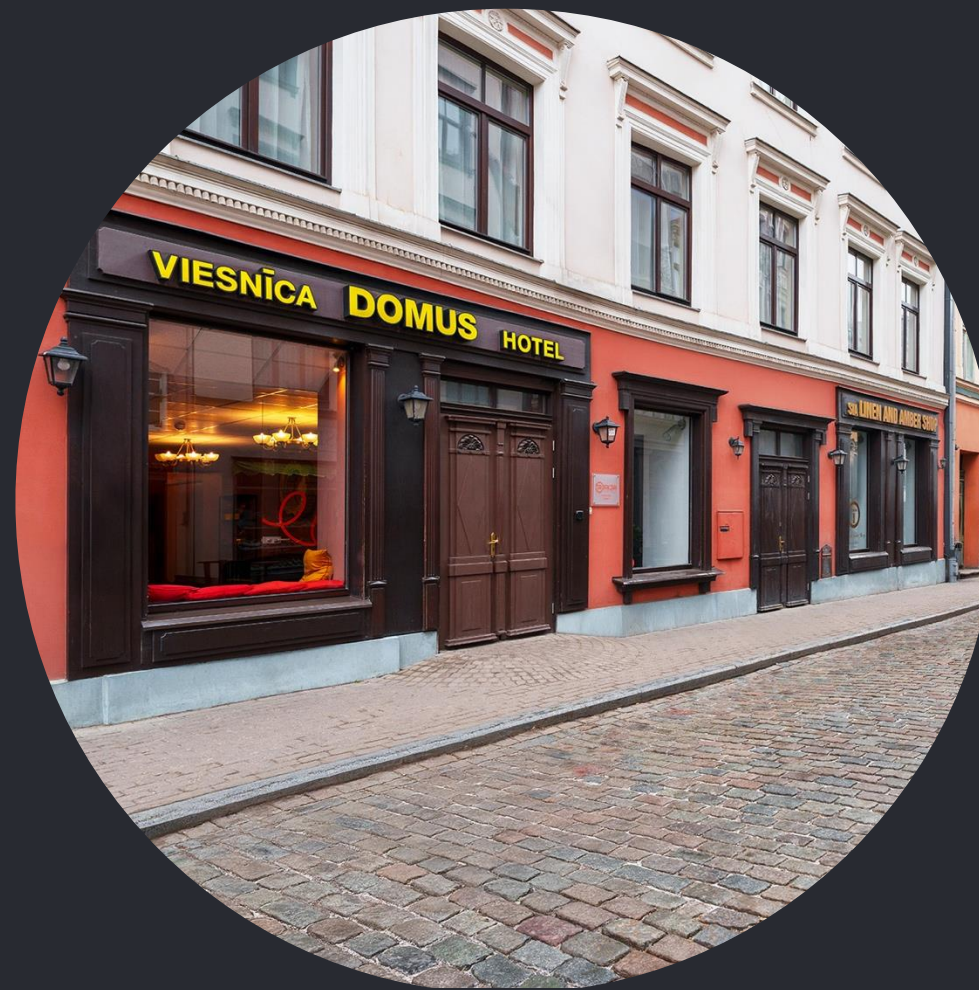
Rija Domus Hotel (under renovation)
